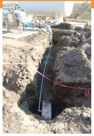
The grower or irrigation company will need to install a 1/2 inch PVC line, from at least one but preferably two elbows downstream of the point of injection of acid. Tap to be on the side.
